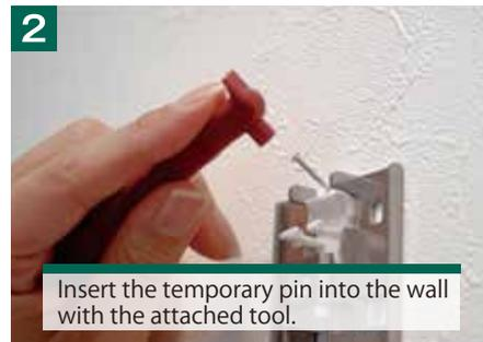
Insert the temporary pin into the wall with the attached tool.
