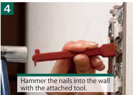
Hammer the nails into the wall with the attached tool.
